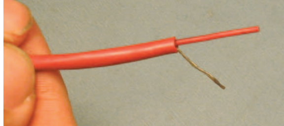
Figure 3.4.14 Ready for connection.
