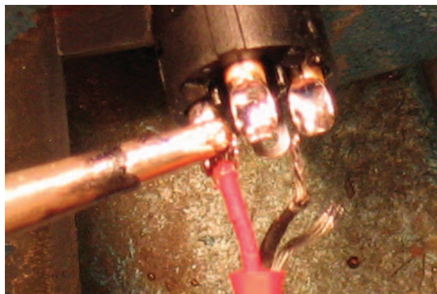
Figure 3.6.28 Attaching high conductor – 2.
